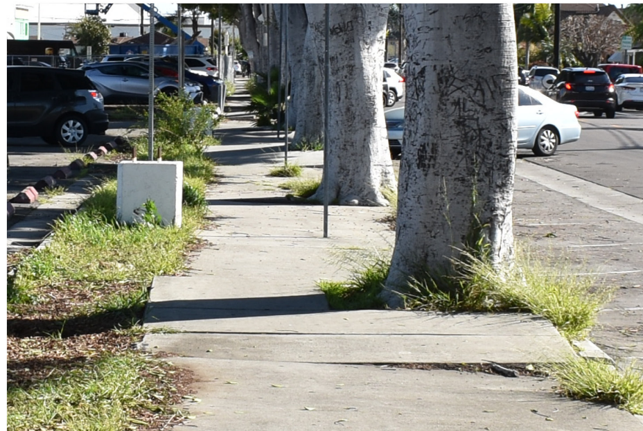
Existing sidewalk condition; located too close to ficus trunks
